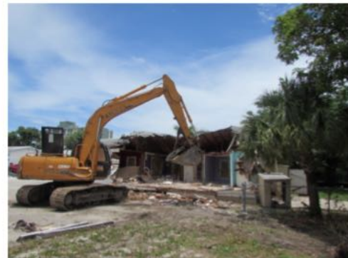
Demolition of the abandoned structures currently on the “A Street Campus” site:
